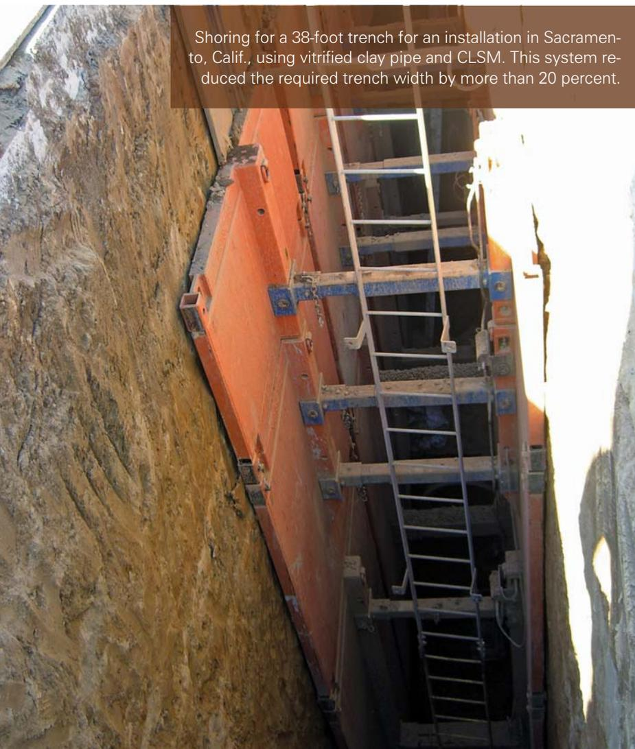
Shoring for a 38-foot trench for an installation in Sacramento, Calif., using vitrified clay pipe and CLSM. This system reduced the required trench width by more than 20 percent.
